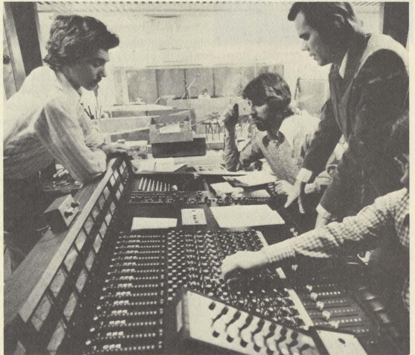
Control Room and Recording Studio
