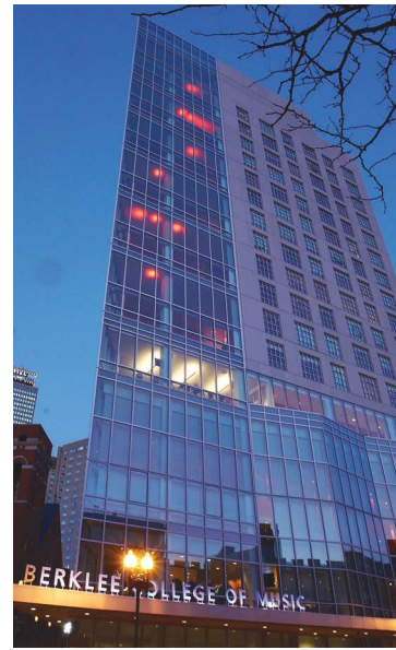
A light show in the windows of the 160 Massachusetts Avenue tower was synced to musical performances.
